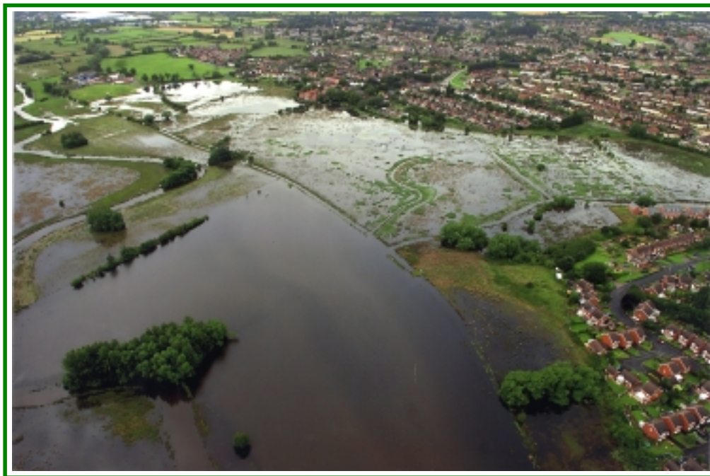
Flooding on the outskirts of Stafford - June 2007
