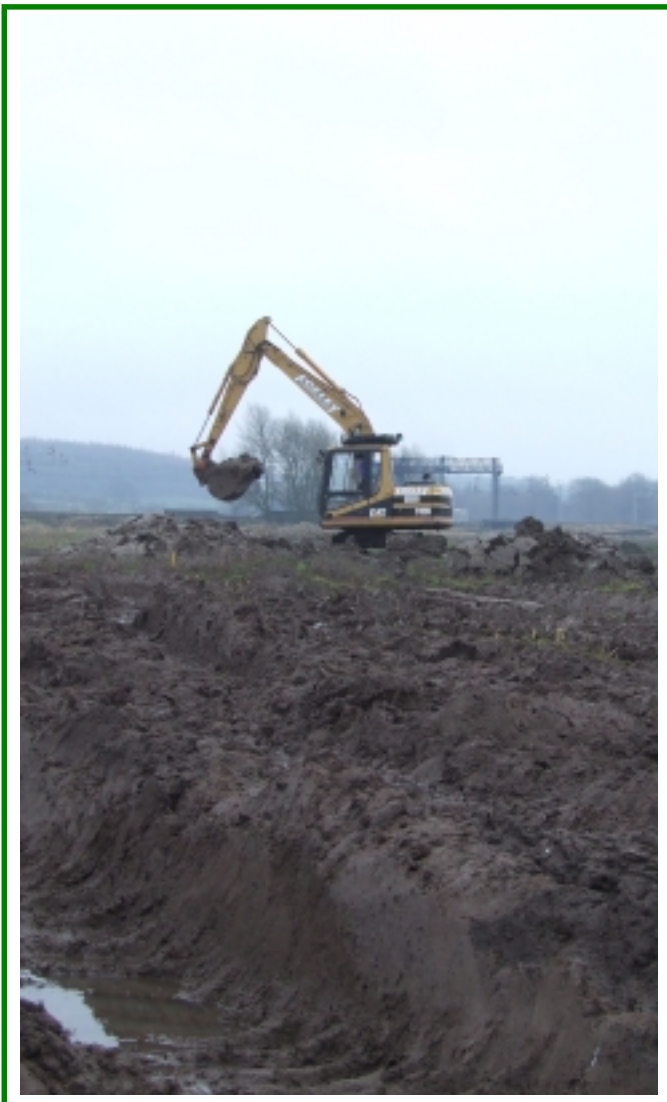
Works in progress at Church House Farm (see Case Study 1)
