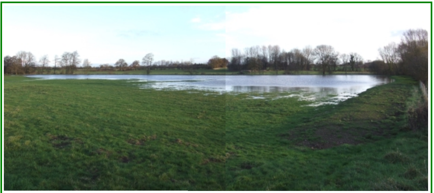
Flood storage scheme in operation at Bellfields Farm (see Case Study 6)
